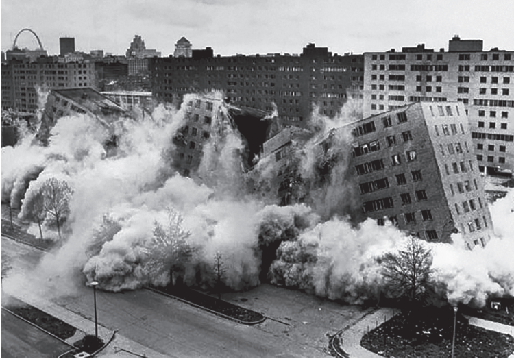
Demolition of Pruitt-Igoe (1972).
