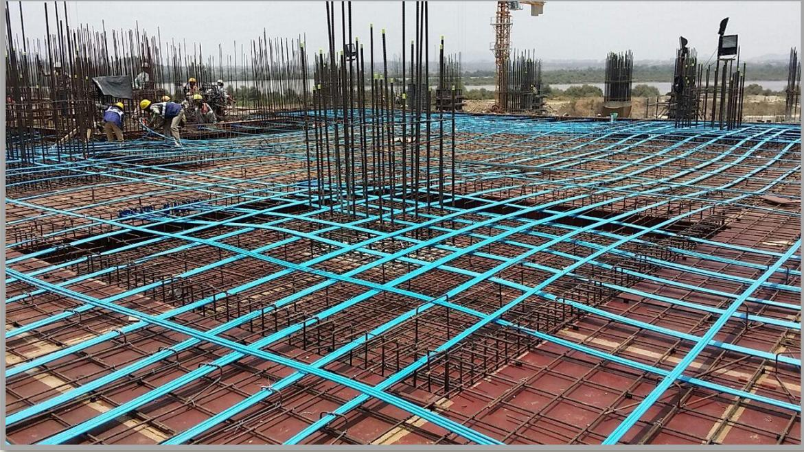
2. Post tensioned in wall of the Tanks
